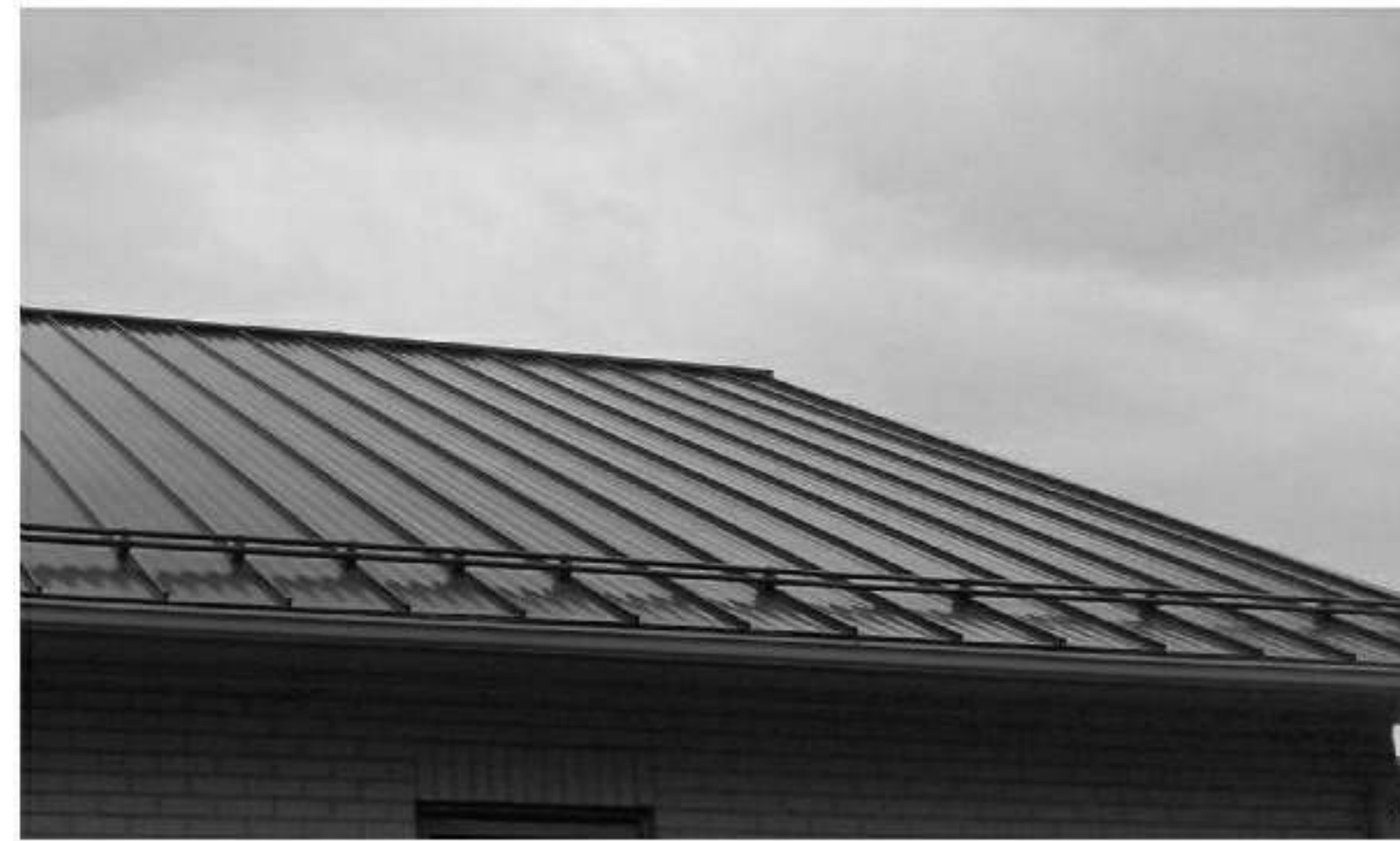
ASG3000G Standing Seam Two-Pipe Snow Guard BASIS OF DESIGN: ALPINE SNOWGUARDS ASG3000G STANDING SEAM TWO-PIPE SNOW GUARD
